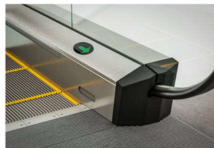
Traveling direction entry sign in green LED.
